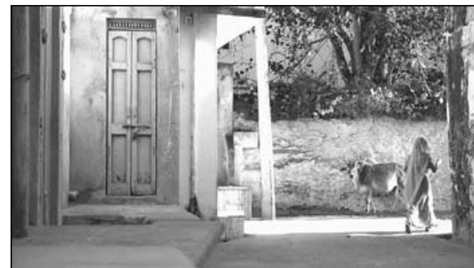
Under the Palace Wall
